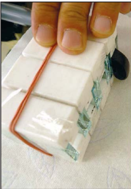
Picture 13: Injection of the silicone adhesive into the joint
