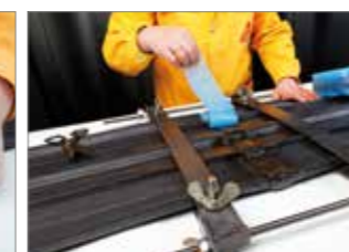
Jointing the waterstop, tightening with the fixing Clamps
