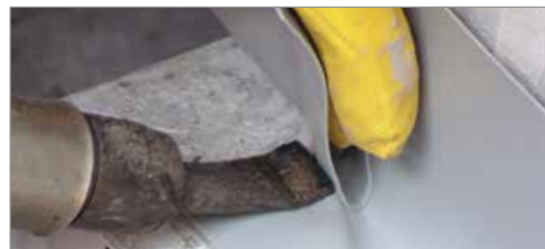
■ 4. Joining membrane strips by heat welding
