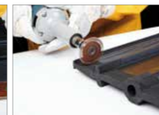
Grinding of the rubber surface
