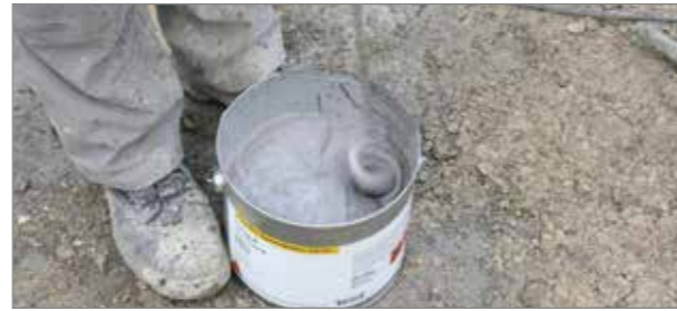
■ 1. Mixing the Tricoflex® FU 60 system adhesive
