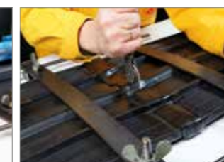
Application of cover strips; pressing home of both cover strips
