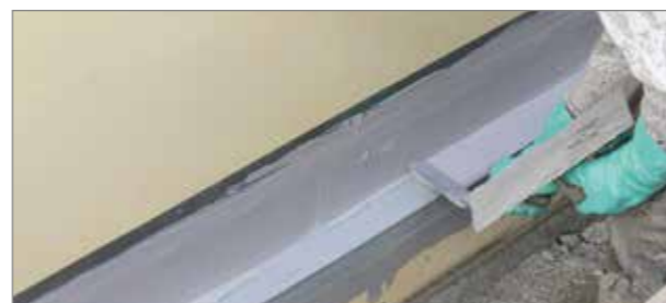
■ 5. Applying the top layer of adhesive
