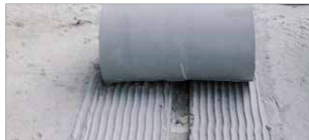
■ 3. Positioning the membrane strip
