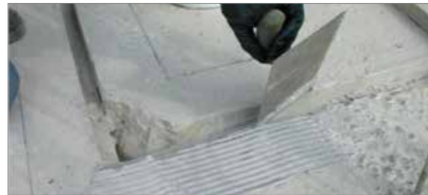
■ 2. Applying the base layer of adhesive
