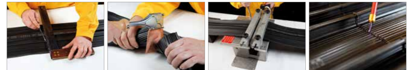
Measuring, marking, cutting
