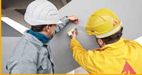
CORROSION AND FIRE PROTECTION
