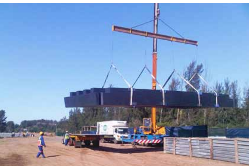
Transporting the pontoons to the coastline
