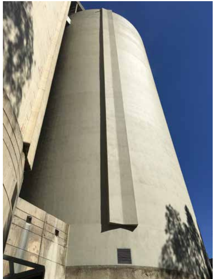
After remedial works.
