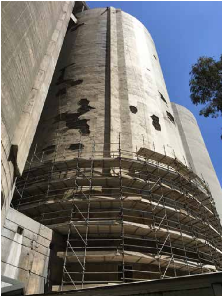
Before remedial works.
